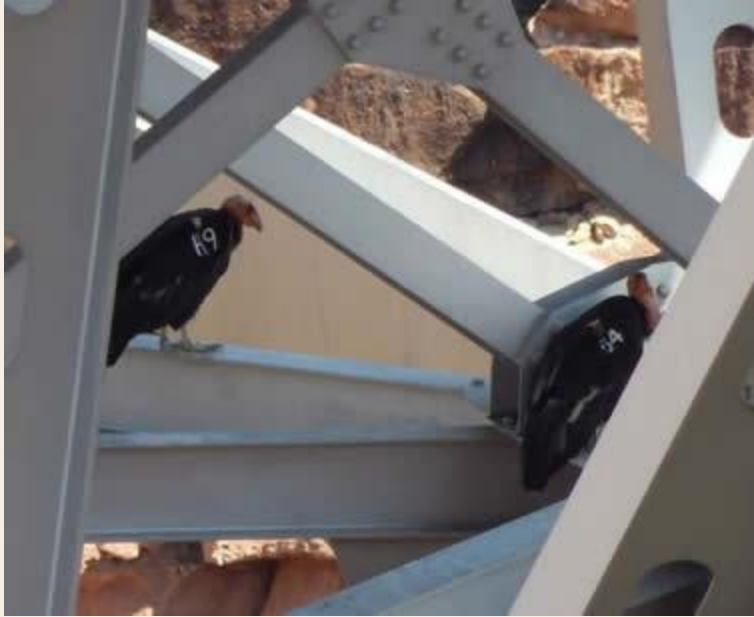
Figure 12. Two of the reintroduced California Condors on the underside of Navajo Bridge (© Eric Hough).
