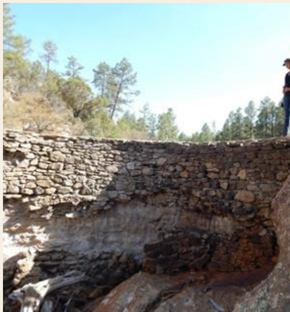
A) Old rock dam at Phillips Tank along White Mule Creek
